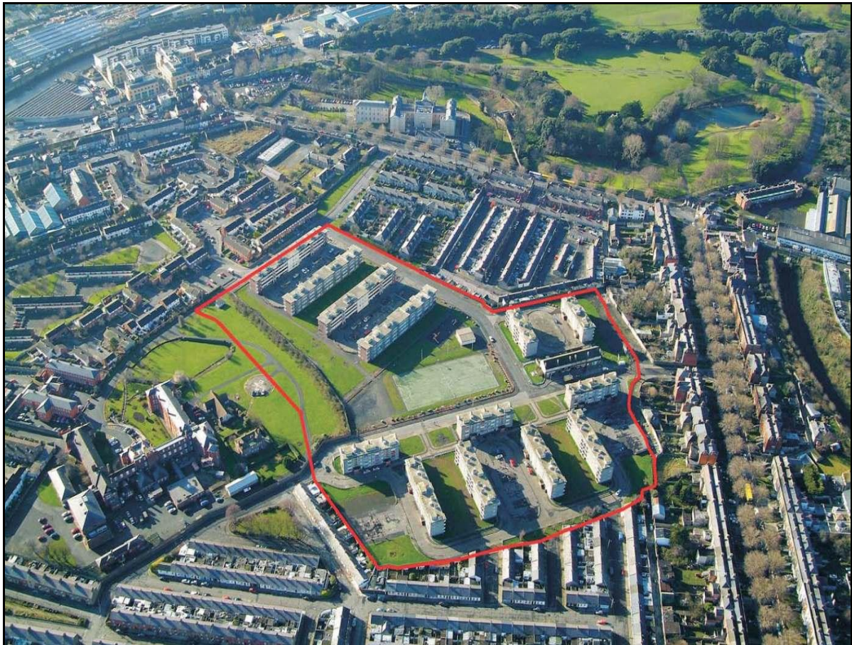
Figure 1: Aerial Photo of former DCC flat complex O'Devaney Gardens.
