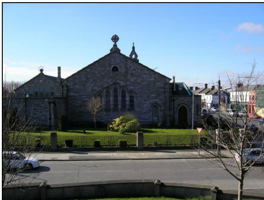
Figure 11: St. Michaels Church (view from Bulfin Road)
