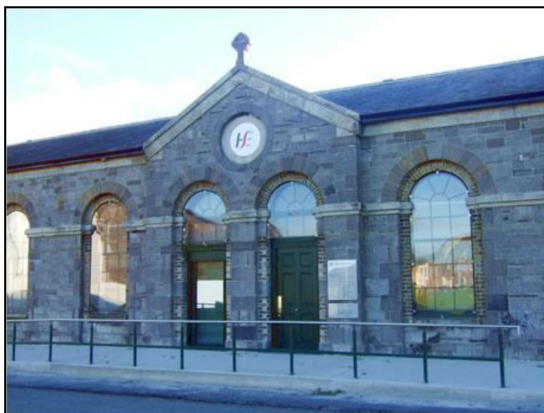
Figure 12: HSE Primary Health Care Centre
